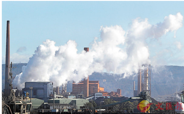
A petrochemical plant
