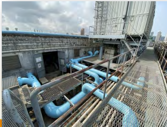
New chiller pipes connected to cooling towers
