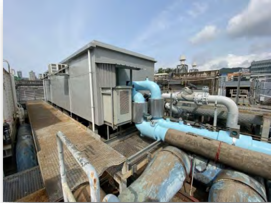
New chiller pipes
