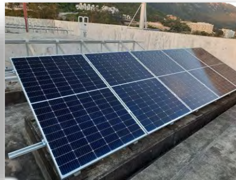
New installed PV Panel
