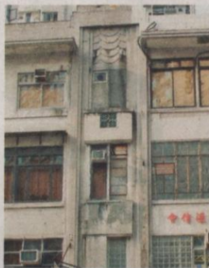
Art deco facade of a block of flats on Prince Edward Road, Kowloon.
