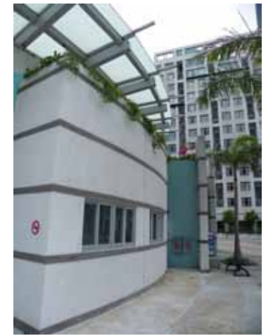
Green roof in the SRO's new office annex: provide insulation and reduce heat island effects.
