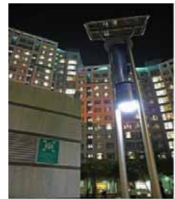
Solar-and-wind light towers: create adequate lighting in the areas by harnessing natural resources without consuming electricity
