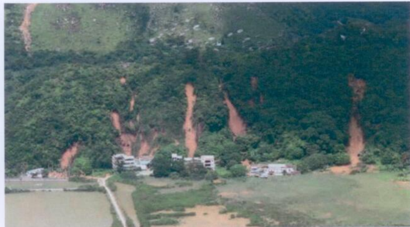
FIGURE III. Some of the 2400 landslides occurring on Lantau Island near Tai O, Hong Kong triggered by the severe June 7 2008 rainstorm. Total rainfall reached a maximum of 384mm over a 4-hour period. Courtesy of the Civil Engineering Development Department, Hong Kong SAR Government.
