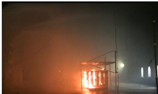
(f) 240 s after activating WFFF system
